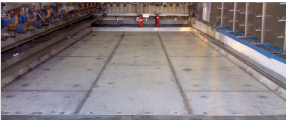
Ground protection lining made of stainless steel
