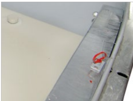
Dipstick to register any leakage
