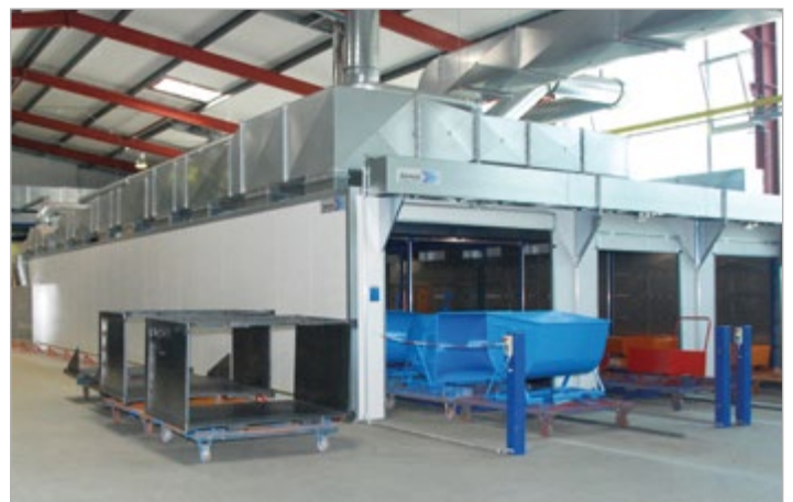
Paint shop with drying street
