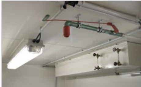
Emergency shower with 250 litre tank and explosion proof lightning
