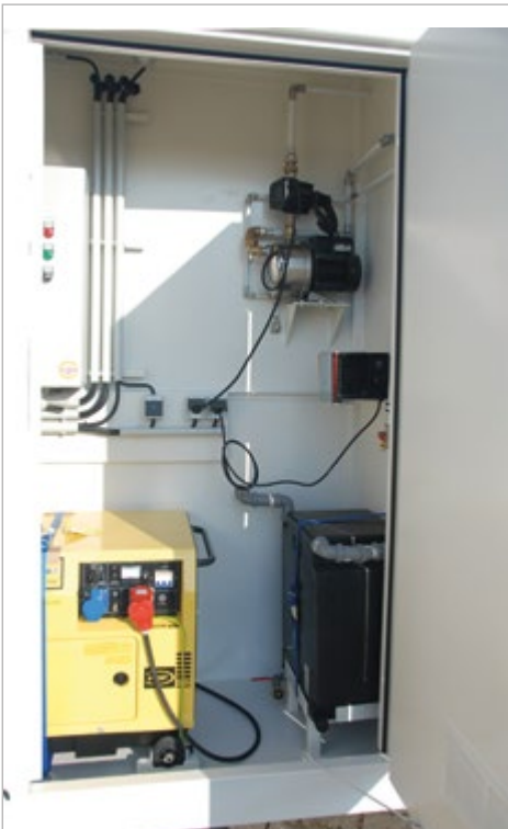
Engineering room with ventilator, switch cabinet and emergency generator
