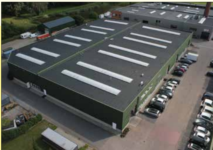
Barendrecht, The Netherlands - Production and Logistics
