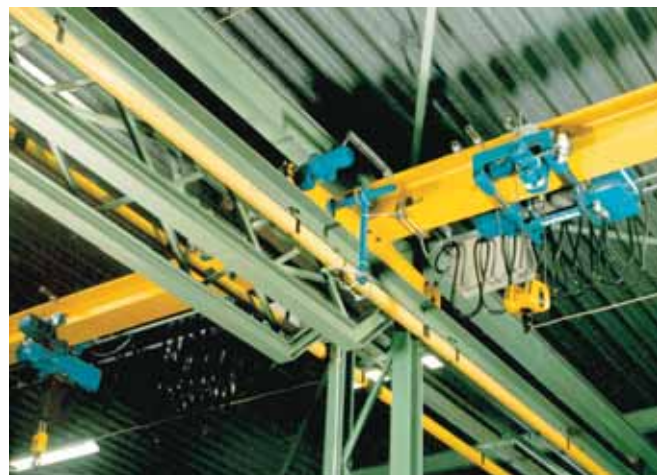
Supply for crane installation
