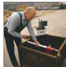
Straightening of a container box by use of a hydraulic cylinder YS-10/100, extension tube AYS-106, base adaptor AYS-103 and electric power pump PY-04/2/5/2 M.
