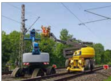
Construction of contact lines
