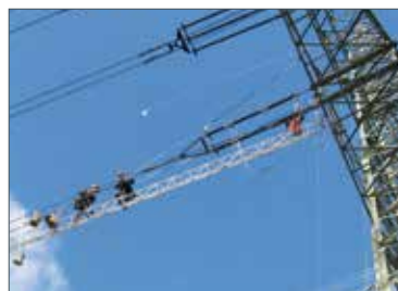
Overhead line construction
