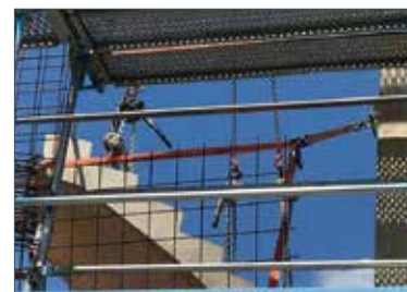
Positioning of loads
