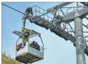
Cable car construction
