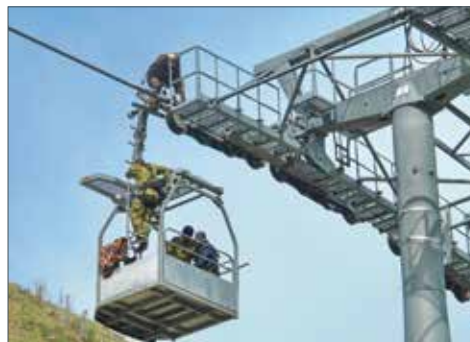
Cable car construction
