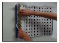
Place filter in frame and tuck each end pleat behind the bent tines.
